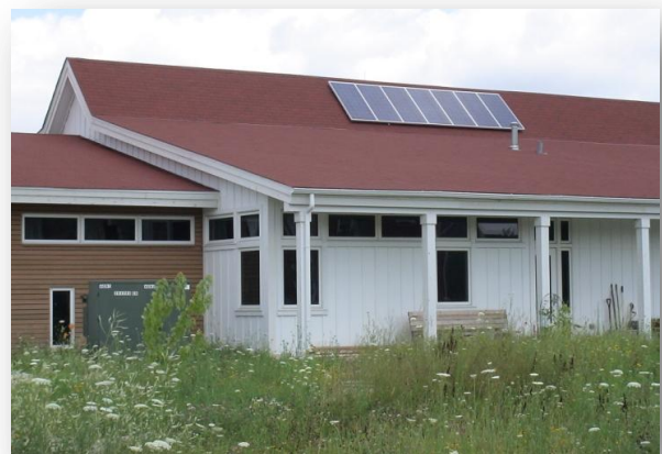
Solar Array on the Prairie Crossing Charter School – USBC-certified LEED Gold.
